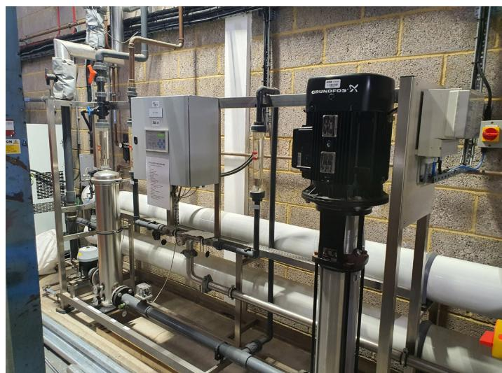
Water softening plant inc: 3x tanks – caustic thermo-tech, phosphate thermo-tech, sulphate thermo tech, each tank with 3x Grundfoss DDC6-10A digital dosing pumps (2016)
