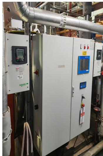
Herco Wassertechnik UO8000ND reverse osmosis plant, 11kW, RO1000 control, FHD 610330AN20C1EED1 filter, Grundfoss 11kW motor / pump, 2660ltr/hr min concentrate flow rate, 8000ltr max permeate flow rate (2016)
